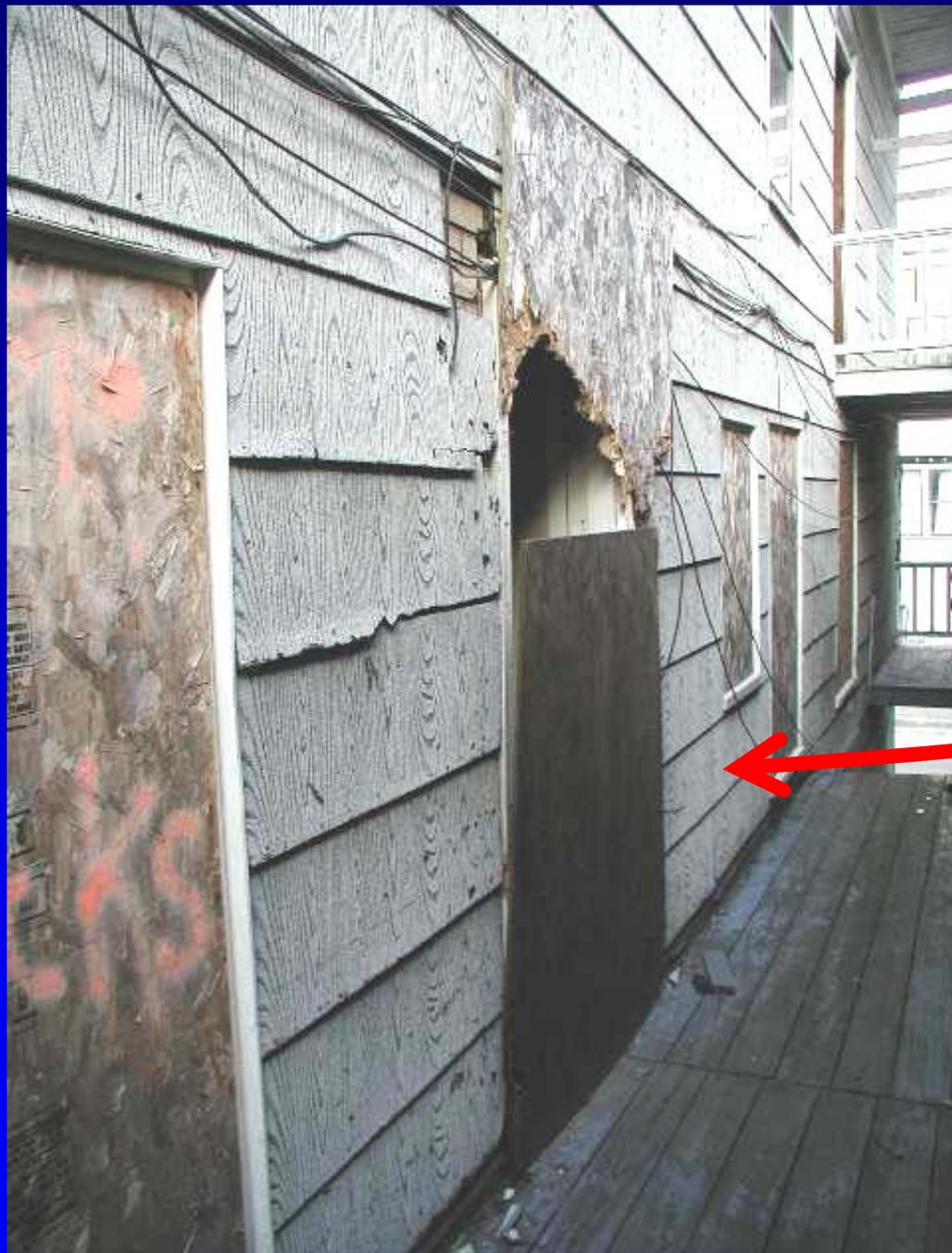
The building was boarded well on street level. On the 2<sup>nd</sup> floor, wood was easily pulled away without tools.
