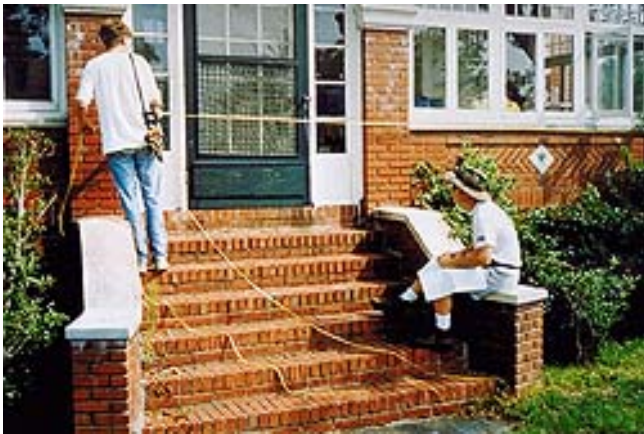
Documenting a building's history and assessing its condition provide information to set priorities for stabilization and repair, prior to mothballing. Photo: NPS files.
