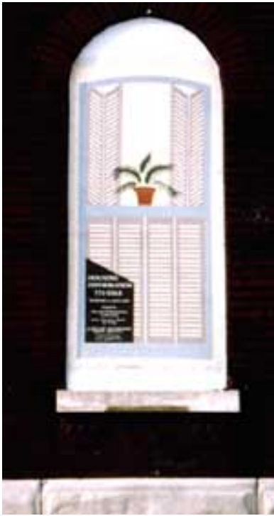
This painted trompe l'oeil scene on plywood panels is a neighborhood-friendly device. Photo: NPS files.
