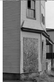
The importance of specifying the use of proper methods and materials is shown on this slide. Communities with no regulations regarding board-up procedures will get this type of work because the materials are the least expensive. Particle board is a very poor choice because it loses its integrity after it gets wet. After a few weeks, a particle board board-up can be easily breached, usually without tools.
