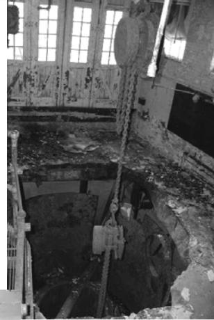
Open shafts, pits and damaged stairways create hazards to anyone entering the building. These openings will also allow the fire to travel rapidly to other parts of the building.
