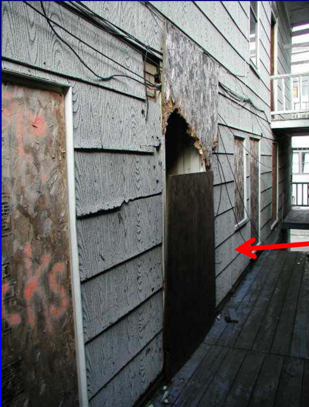
**The building was boarded well on street level. On the 2<sup>nd</sup> floor, wood was easily pulled away without tools.**
