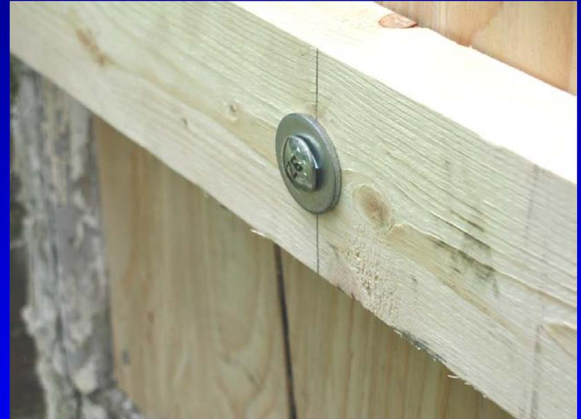
**Monitor installation and avoid pry points on braces and bolt assemblies**
