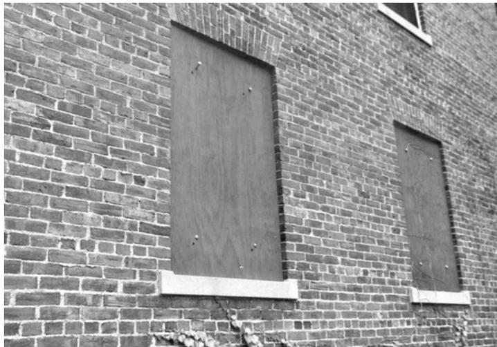
The HUD board up procedure uses plywood covers for window and door openings that are held in place using carriage bolts and 2 x 4 braces on the interior. While it is more secure than plywood attached to windows or doors with nails or deck screws, it can be breached by driving the bolt through the plywood.
