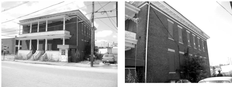
This slide shows an example of a non-reinforced board-up of a historic structure. Note vents and light panels on upper floors. This is the least complex and lowest cost method for securing a structure. It is also the easiest to breach.
