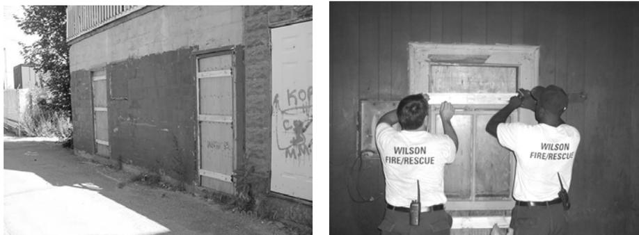
This method is the method of choice for high threat locations. It is the most secure type of board-up and also the most costly. The installation for windows and doors is discussed in more detail later in the program.
