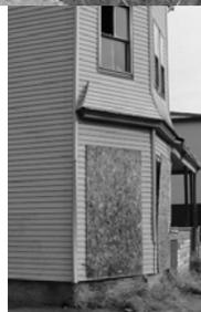
This slide shows the importance of doing the job well with the proper materials. Particle board is ineffective as a security measure. It deteriorates rapidly when exposed to weather and is easily breached by anyone who wants to gain access to the building.
