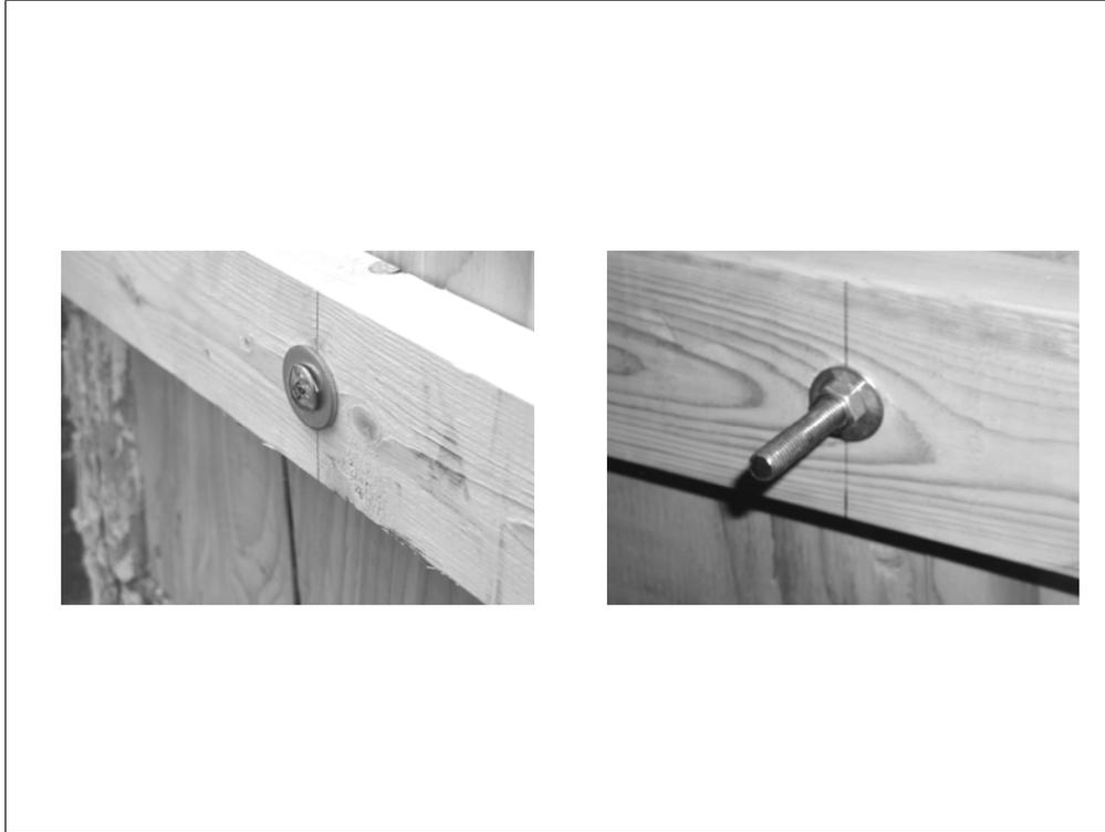
Interior and exterior photos of the carriage bolt assembly are shown. Avoid pry points on the outside surfaces as shown on the left slide.
