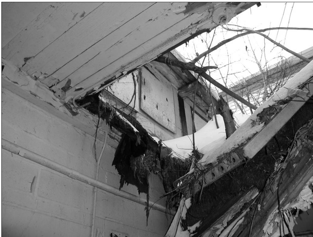
Snow loading and water deterioration affecting integrity.
