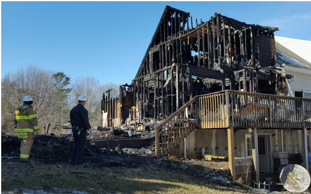
Credit: Bedford County (VA) Fire Marshal's Office
