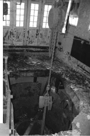
Fall and trip hazards are common problems in vacant/abandoned buildings. These hazards may be the result of equipment removal, urban mining ( the removal of items of value by vandals), or vandalism as in the removal of stairs or stair railings. In some instances, holes are purposely cut into floors in an attempt to cause injury to those entering the building – including fire fighters.
