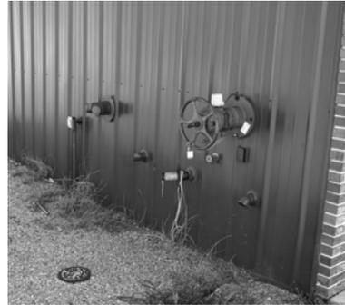
Determine the operational readiness of any installed systems. If a building is provided with a sprinkler system, is the piping intact even though it may be drained with the valves off? Where piping is intact, there may be an option to feed the system via the fire department connection in the event of a fire. Point out the ice coming from the 2 inch drain valve in the photo above.
