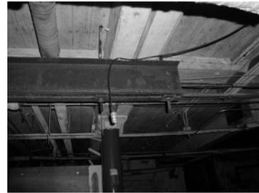
Where structural components are exposed, either by design or as a result of deterioration or vandalism, they will be exposed very early in the progression of a fire in the structure. This is also an indicator that structural failure and collapse could occur early in the development of a fire in the building.
