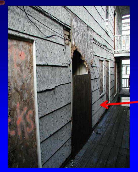
The building was boarded well on street level. On the 2<sup>nd</sup> floor, wood was easily pulled away without tools.
