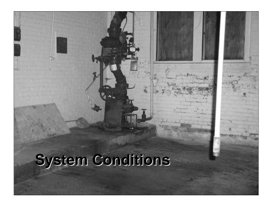
Consider shut valves (zones) broken and scavenged piping. If piping is intact, can it be used to assist in fire control?
