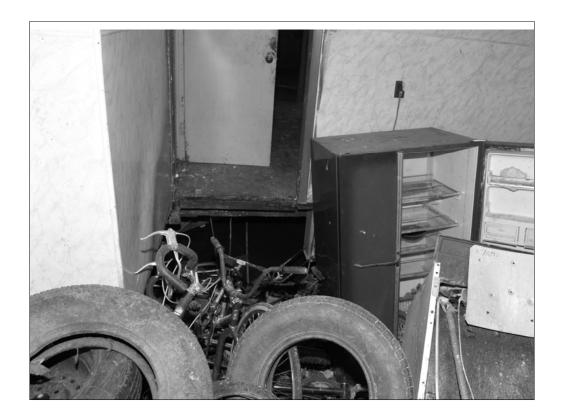
Point out collapsed floor, tires and trash that could entangle a firefighter working in heavy smoke.
