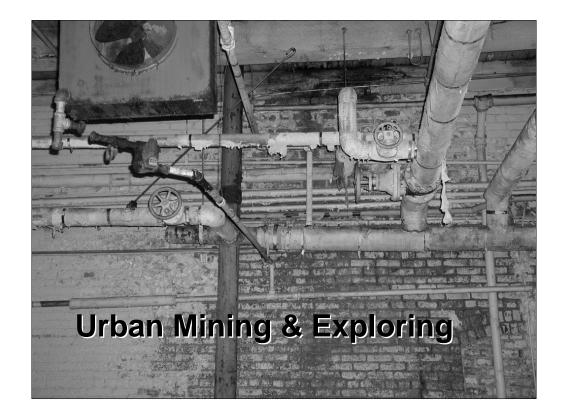
Piping, electrical wiring, and other materials of value may be removed. What will be left behind will be asbestos, openings, void spaces etc.
