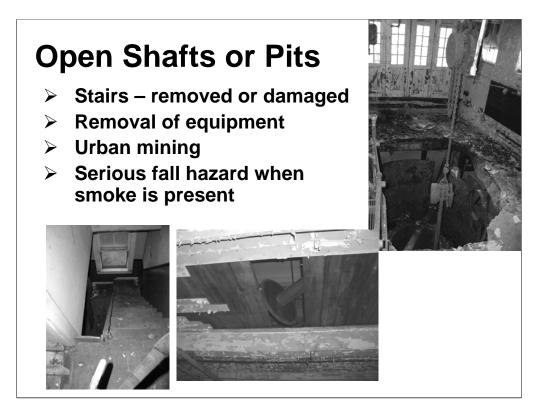
Open shafts, pits and damaged stairways create hazards to anyone entering the building. These openings will also allow the fire to travel rapidly to other parts of the building.
