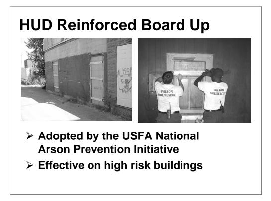
The HUD reinforced method, also known as the USFA National Arson Prevention Initiative method, is the method of choice for high threat locations. It is the most secure type of board-up and also the most costly. 2 x 4 braces on both sides of the opening are compressed using 12-inch carriage bolts. This method requires significant effort to gain access when properly installed.
