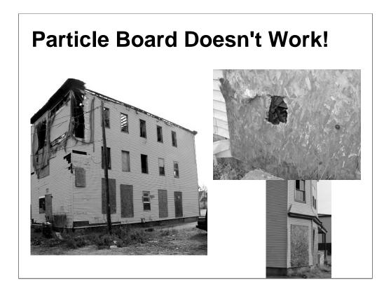
This slide shows the importance of doing the job well with the proper materials. Particle board is ineffective as a security measure. It deteriorates rapidly when exposed to weather and is easily breached by anyone who wants to gain access to the building.
