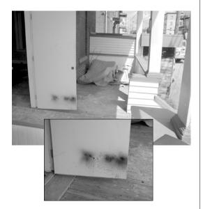
Note that the door in this photo has a hole through it for placement of a door knob. This opening has been used to drop fireworks or burning combustibles into the building. Doors used for this purpose should be without openings, or they should be securely covered when installed.
