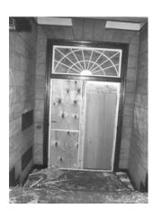
Discuss the method for dealing with large openings. Many times a 2 x 4 frame will have to be constructed and the plywood and braces attached to the frame and building. For openings that the through-bolt compression method is not practical, the opening should be covered using plywood that is secured to the structure using 3-inch wood screws applied on 4-inch centers around the circumference of the opening.
