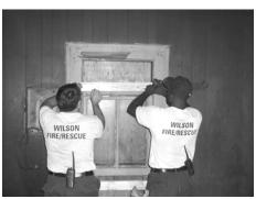
This method is the method of choice for high threat locations. It is the most secure type of board-up and also the most costly. The installation for windows and doors is discussed in more detail later in the program.
