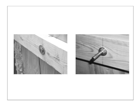
Interior and exterior photos of the carriage bolt assembly are shown. Avoid pry points on the outside surfaces as shown on the left slide.
