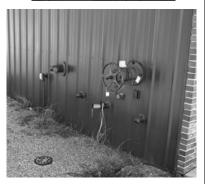
Determine the operational readiness of any installed systems. If a building is provided with a sprinkler system, is the piping intact even though it may be drained with the valves off? Where piping is intact, there may be an option to feed the system via the fire department connection in the event of a fire. Point out the ice coming from the 2 inch drain valve in the photo above.
