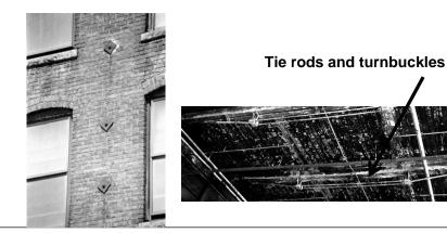
Cracks in exterior walls are an indicator that the wall is deteriorating. Stars or plates on the exterior are an indicator that metal tie rods have been installed in the building to assist in stabilizing the walls. This system is very sensitive to increased heat. The rods lose strength when the temperature approaches 1100°F. When this occurs the walls no longer have the support they were intended to have from the system, thus increasing the potential for wall collapse.
