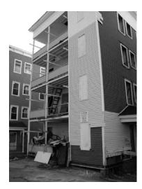
Trash accumulations on the exterior of structures are simple to ignite. This fuel package would more than likely result in a significant fire that extends to the entire structure. This is the type of finding that requires immediate attention.
