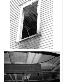
Where structural components are exposed, either by design of as a result of deterioration or vandalism, they will be exposed very early in the progression of a fire in the structure. This is also an indicator that structural failure and collapse could occur early in the development of a fire in the building.
