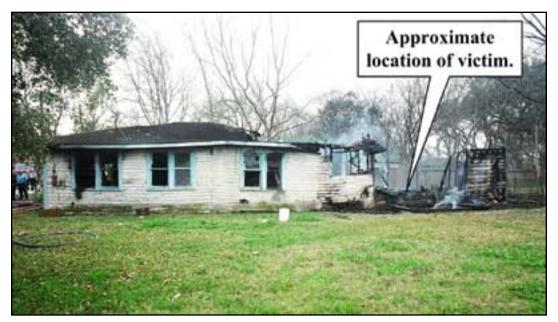
Photo 3. Note roof collapse area at rear of house.
